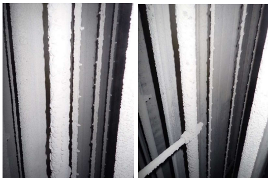
Picture 12 - Ash deposits on collecting and discharge electrodes
