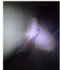
Picture 6 - Boiler ash injection into inlet duct to Main ESP
